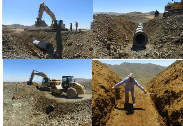
**Figure 7.** The installation process of the culverts
